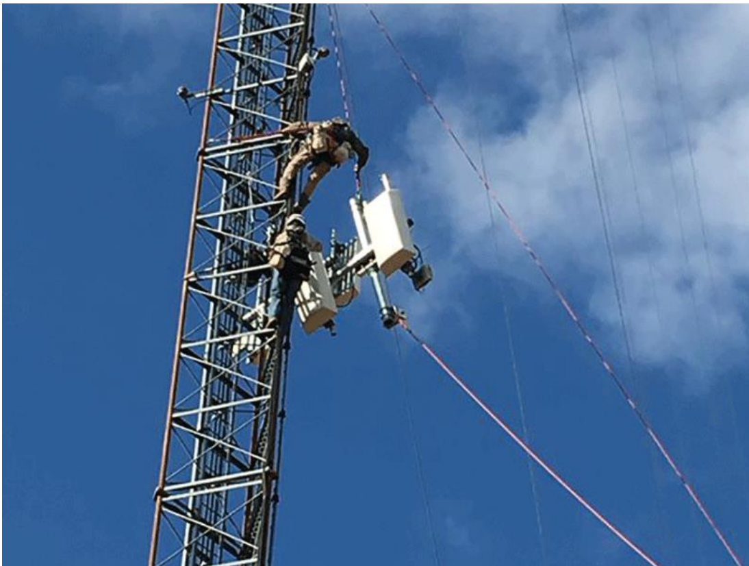
Figure 2: Engineers install TV white space antennas and radios on a tower
