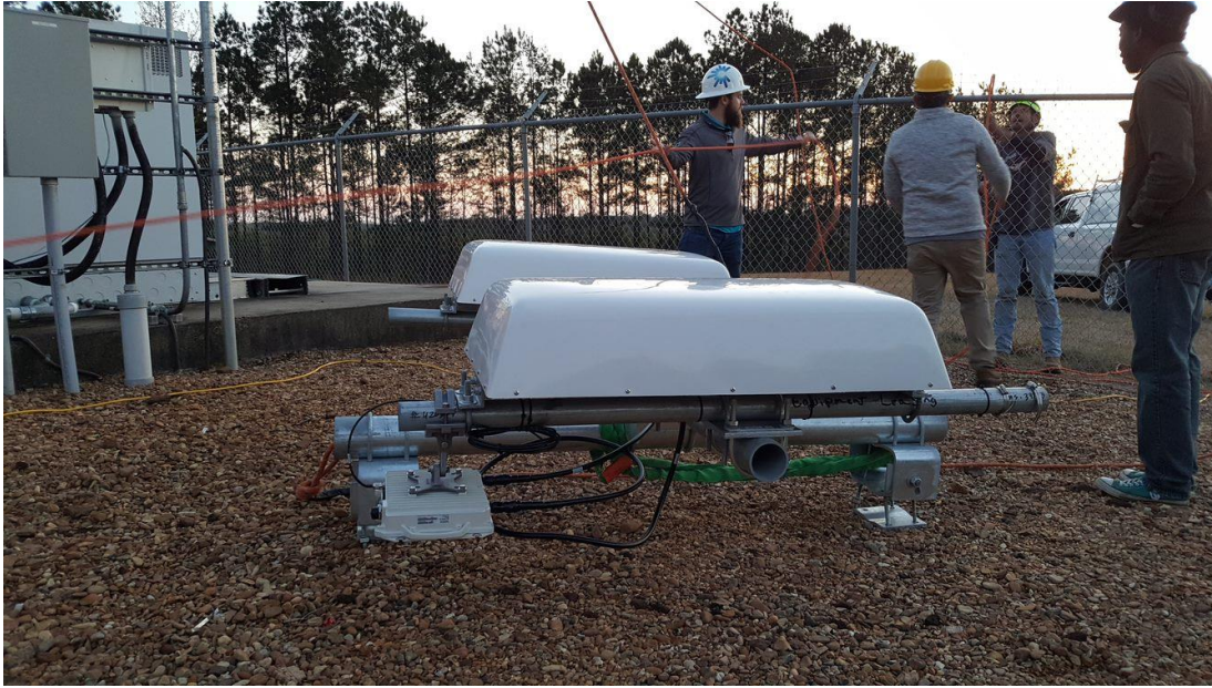
Figure 1: Engineers prep TV white spaces antennas and radios on ground before installation
